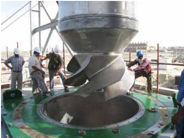
**Super duplex stainless steel fabricated vertical pump**
